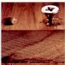
Double fastening of all teak parts for added reinforcement.
